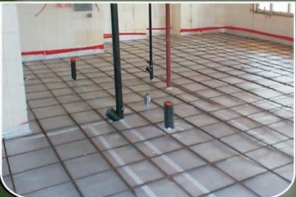
rFOIL<sup>™</sup> Standard and Ultra Concrete Underpad are an outstanding reflective insulation and puncture-resistant vapor barrier. They are composed of a double layer of high-strength polyethylene bubbles sandwiched between one layer of metalized foil, and a layer of clear polyethylene.
