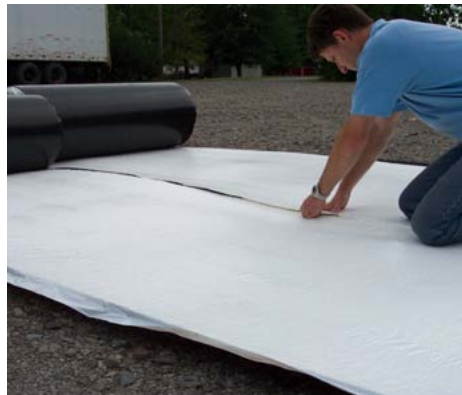
LAY DOWN TUBING / SEAL AROUND OPENINGS
