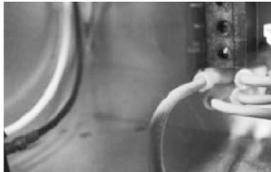
8. Connect red wire from flow switch to boiler wire harness.
